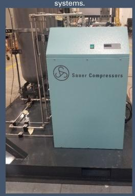
*Figure 1: Sauer USA refrigerated dryer capable of operation up to 6000 psi.*
