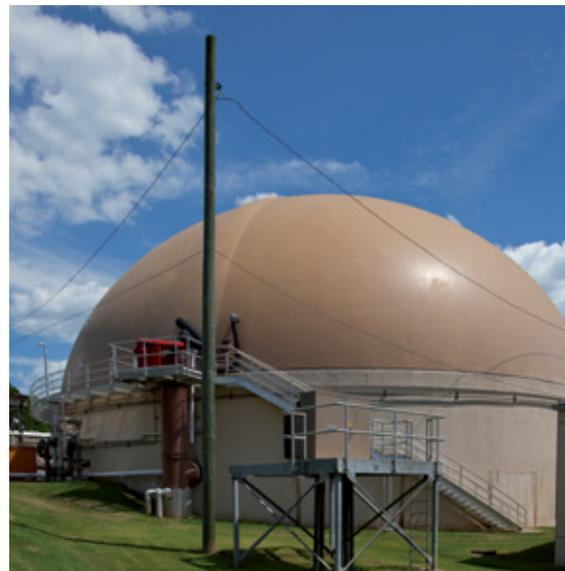
Anaerobic digester producing biogas
