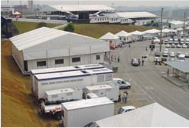
A total of 20 Cummins Rental Power mobile units were used, ranging in size from 100 kW to 1000 kW. The combined power system made available 4 MW of power — enough power to supply a city of 20,000 inhabitants.
