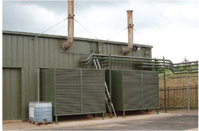
The conduit coming out of the power building contains the 11 kV transmission line that powers the cement plant.
