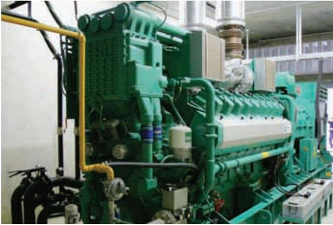
The port's on-site system consists of three 1750GQP lean-burn natural gas generators with a total generating capacity of 5.25 MW.
