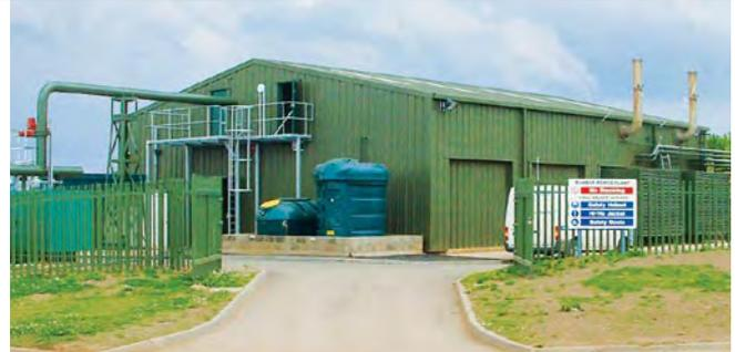
Cummins Power Generation provided a turnkey power system including generator sets with switch-gear and paralleling controls, fuel treatment for the landfill gas, mechanical and electrical design and the power plant building. The two 1750 kW generator sets operate in parallel.
